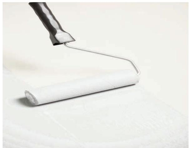
The quantity of material used per coat and the number of coats may vary dependant on the porosity of the substrate and the surface profile.
